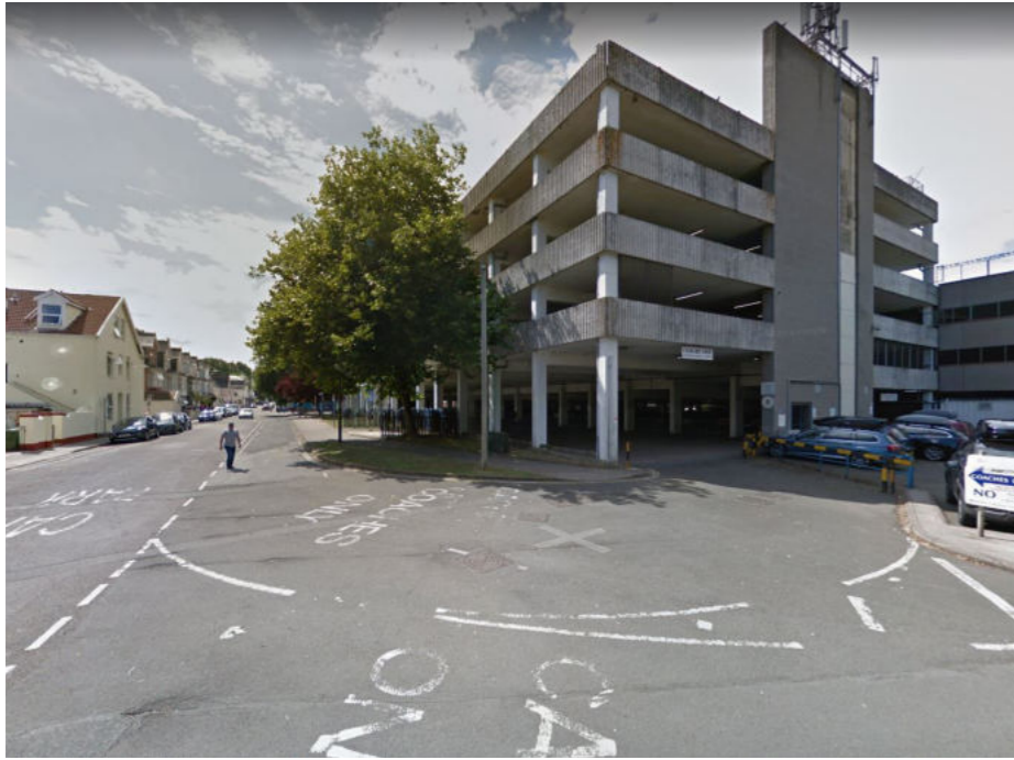
PHOTO 03: View south down Garfield Road
