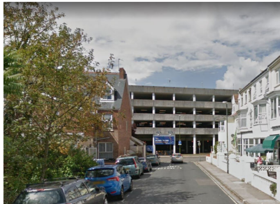
PHOTO 02: View west along Beach Road
